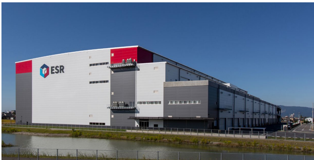
ESR Aisai Distribution Centre is located in the metropolitan Nagoya area, providing tenants with the utmost convenience in transportation and connectivity
