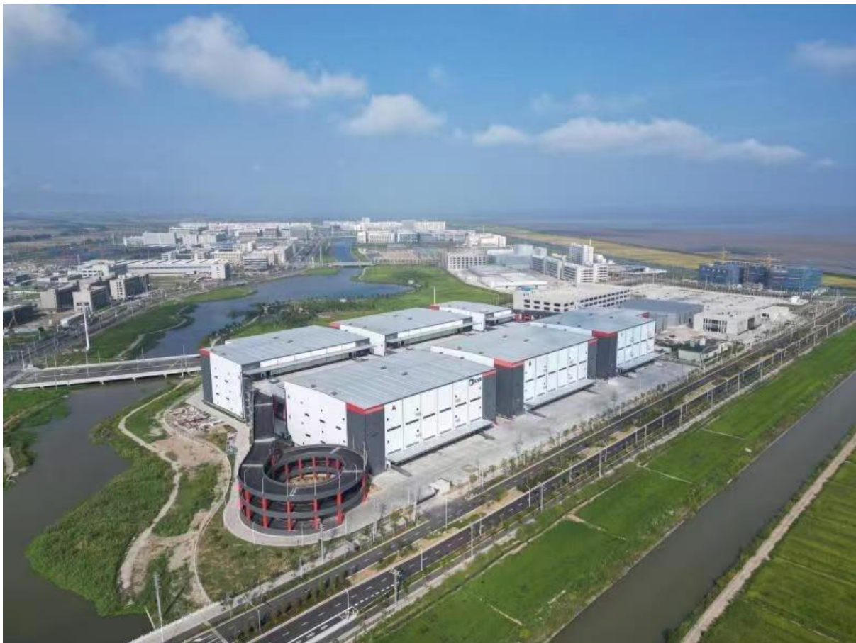
The completed Wenzhou Ruian Logistics Park
