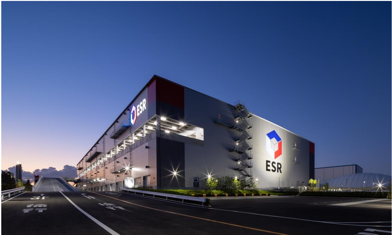
The completed Kawasaki Ukishima Distribution Centre
